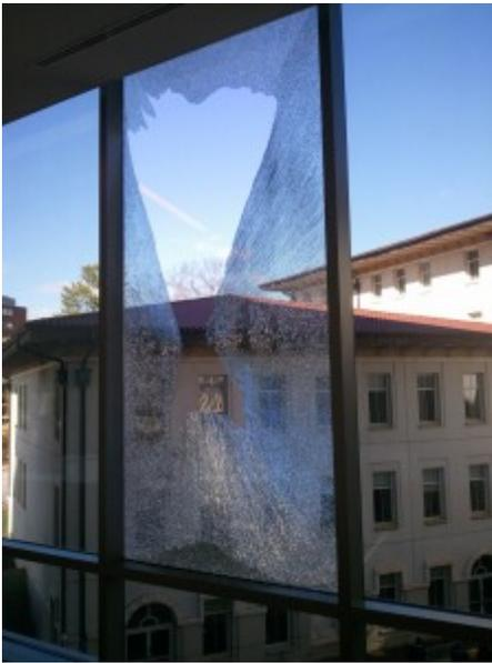
With an increase in spontaneous glass breakage incidents, the glazing industry is looking at new ways to make assemblies safer.
