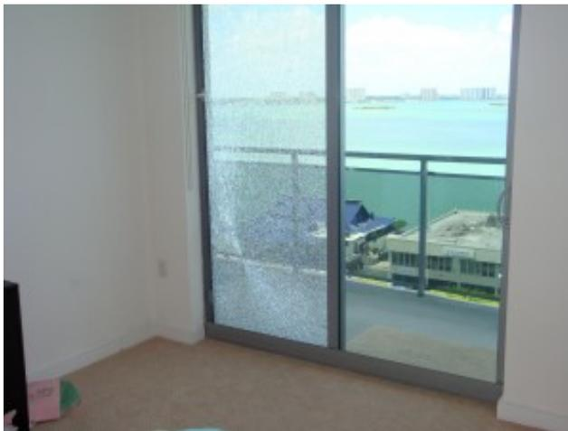
Safety glazings are commonly required for sliding glass doors, shower doors, and patio furniture. 'Safety glazing' generally refers to any type of glass that is engineered to reduce the potential for serious injury.
